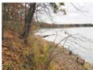
STEEP BANKS AND ERODING SHORELINE
