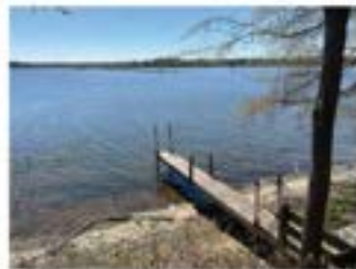
FISHING PIER STRUCTURE
