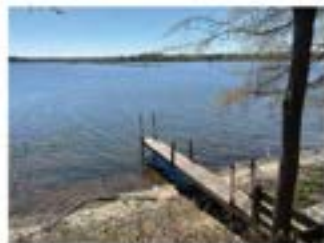
FISHING PIER STRUCTURE
