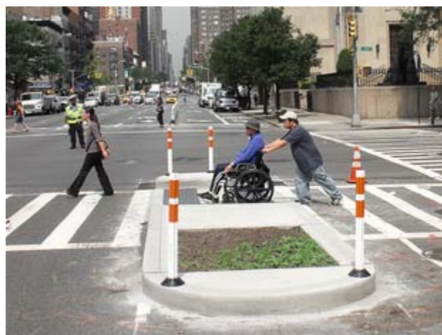
Pedestrian Refuge Island allows pedestrians to cross only half of the roadway at a time. Source: Flickr
