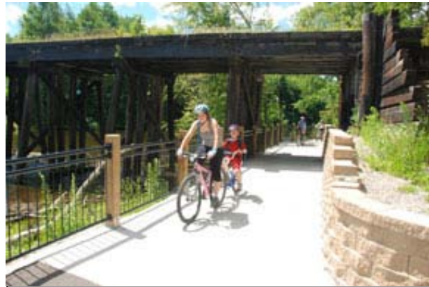
Non-motorized transportation provides a means for people of all ages to access community assets
