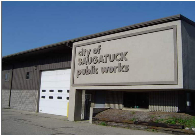
Photo 6-8 Saugatuck Public Works Department Building
