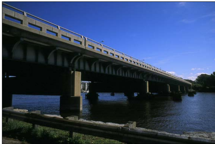
Photo 8-2 Blue Star Highway Bridge
